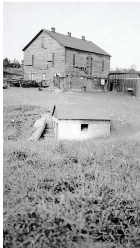
2. View of the Froebe barn in 1917 with the springhouse in the foreground.
