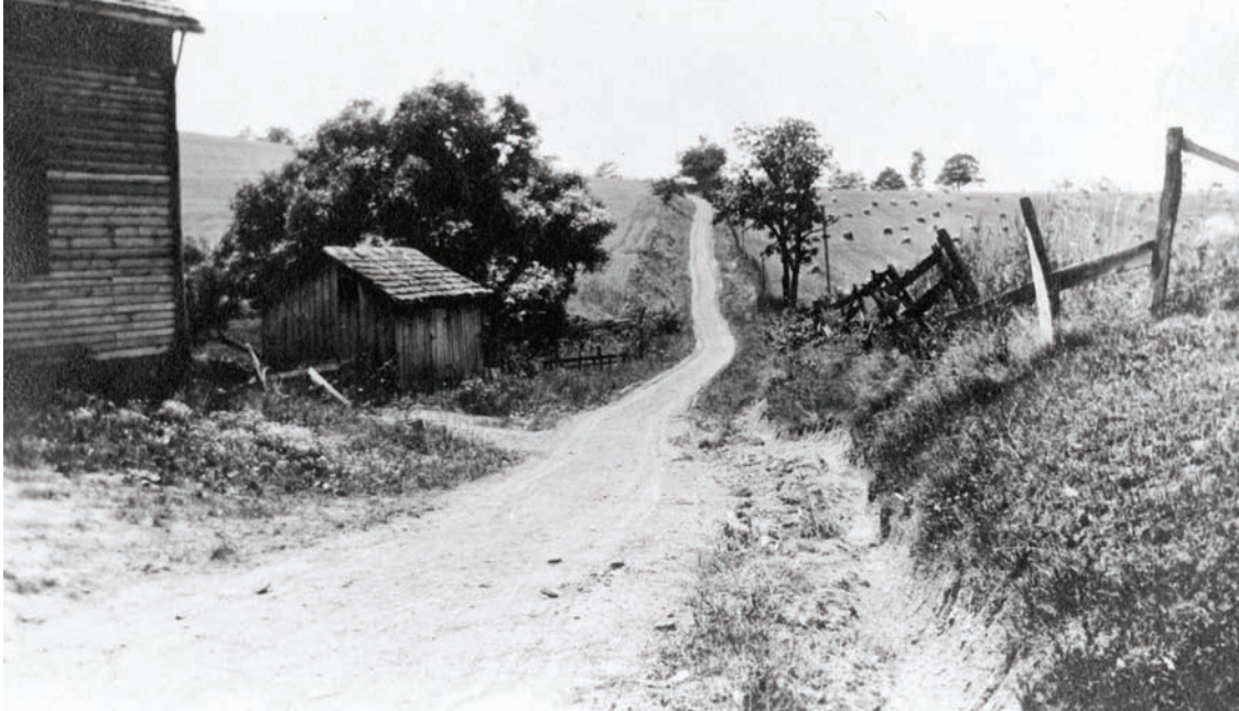
10. Froebe Road before it was widened.
